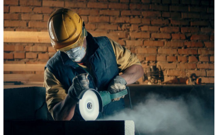
Figure 1, Construction worker demonstrating correct usage of disposable respirator
